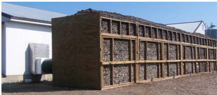
Researchers at the University of Minnesota have tested a vertical biofilter that treats exhaust air from a commercial-type pig nursery barn. Exhaust air flows from the barn through ducts and then into a tall, packed bed of living material that biologically degrades the pollutants in the exhaust air. Photo by Larry Jacobson, University of Minnesota.
